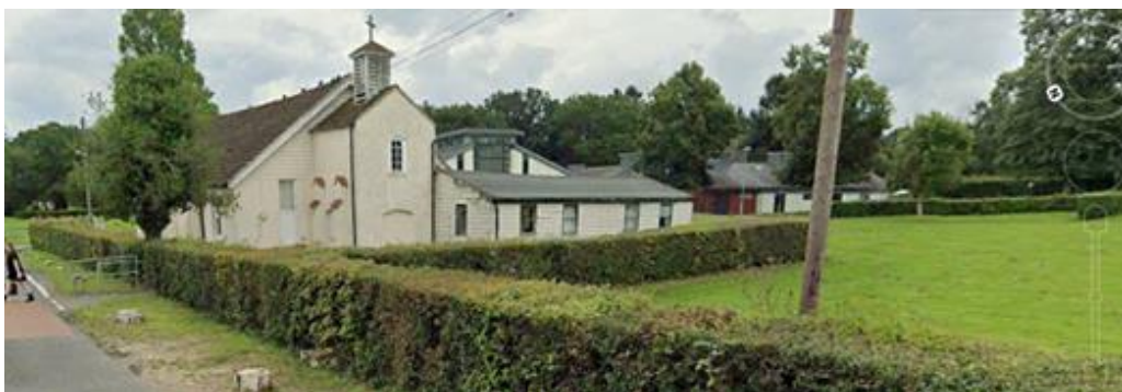
Fig 6. The chapel to the south of St Piers Lane
